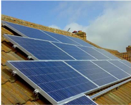
Figure 1: Typical Photovoltaic Arrangement
